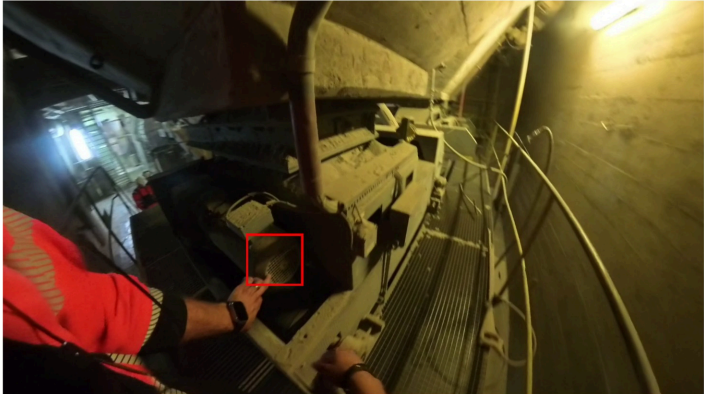
Clean Geared Motor and Check Fan on 535-DB1
