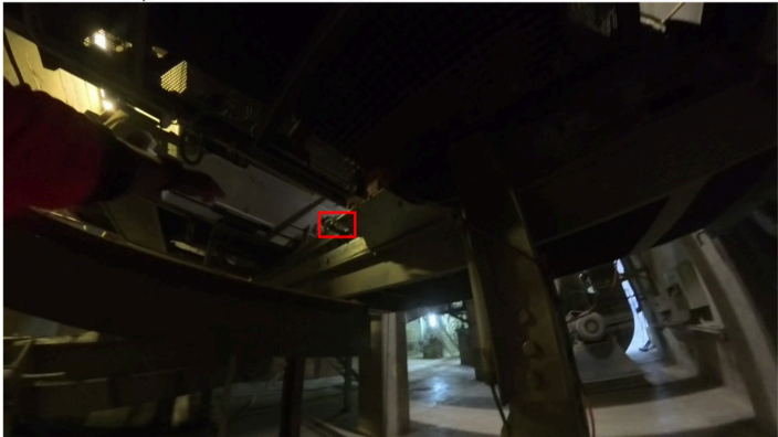
Inspect Pull Wire Switch on Belt 535-DB5
