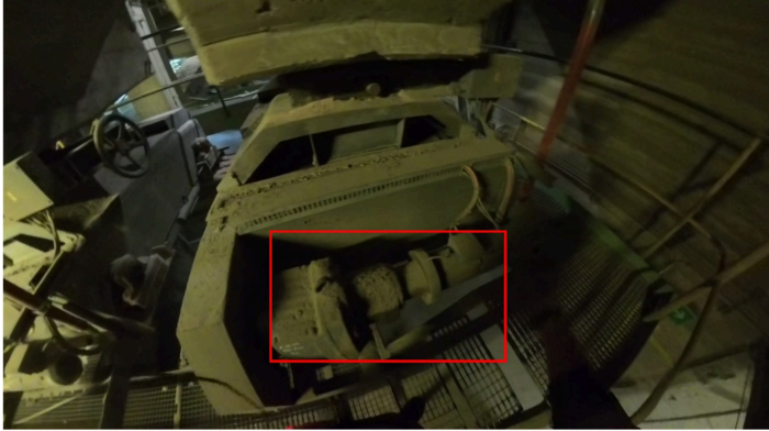
Inspect Bearings and Motor on Limestone Belt 535-DB3
