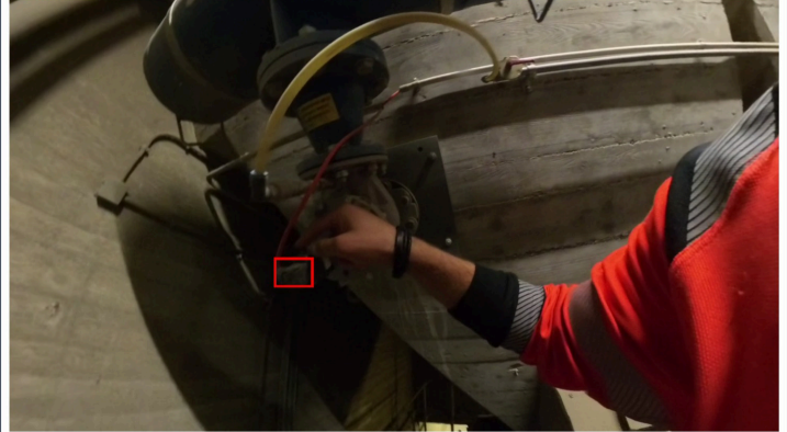
Test Fire Bunker Air Cannon Manually
