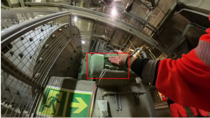
Check Lube Pump 565-SM2 and Motor Temperature
