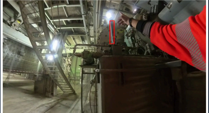
Inspect Oil Filter Clogging Sensor
