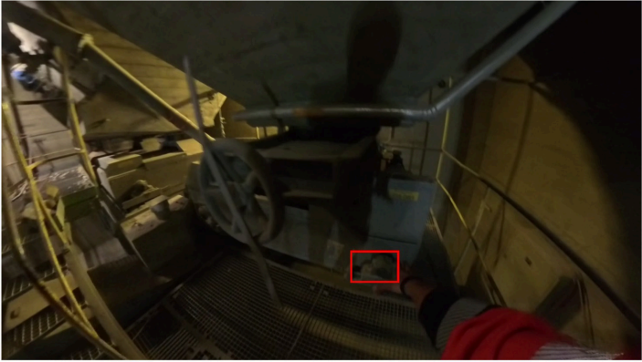
Inspect Bearings on Clinker Belt 535-DB1
